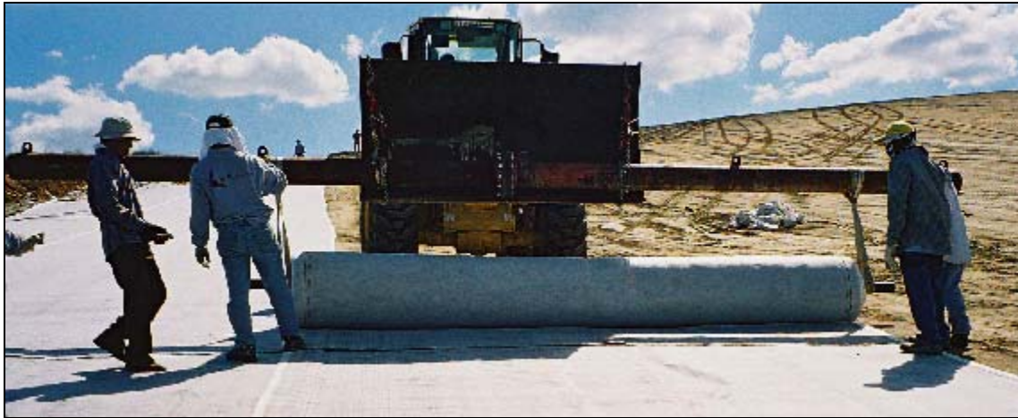
Figure 6. Typical means of liner deployment, using a backwards-moving front-end loader.
