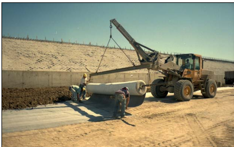
Figure 1. Deployment of the liner using core pipe and spreader bar.
