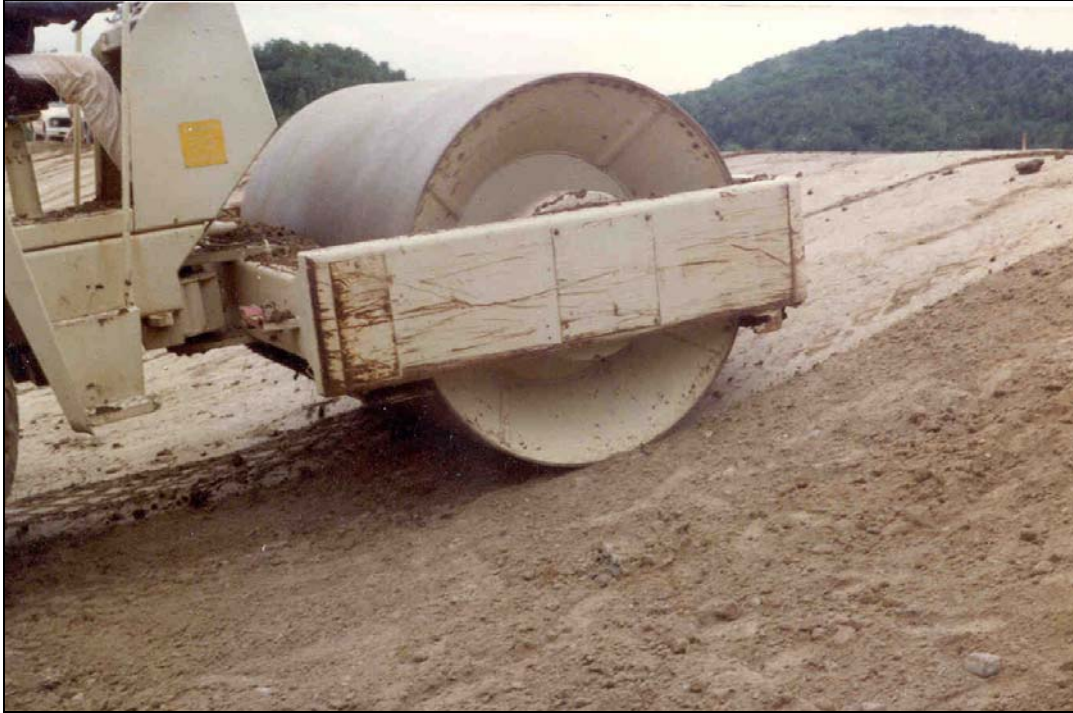
Figure 4. Use of a smooth-drum compactor for subgrade preparation.
