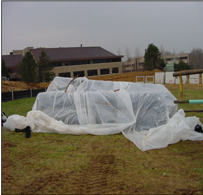
Figure 3. Proper storage of Akwaseal on site.
