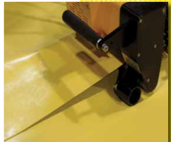
Automated Field Welding
